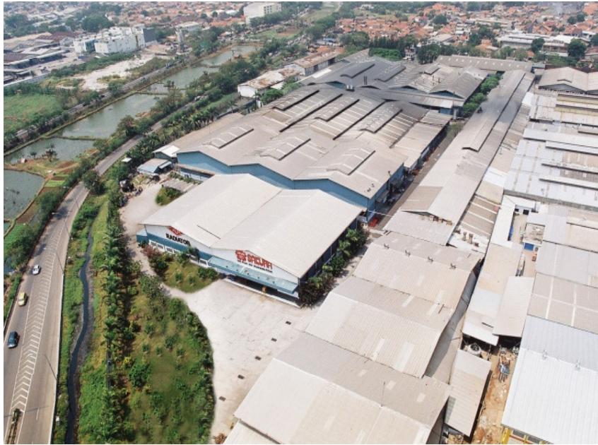
Kapuk Plant (Radiator Facilities)
